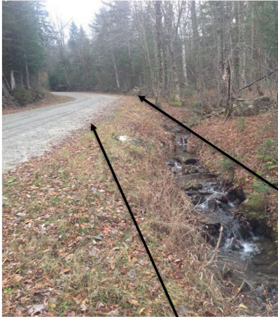
Figure 5: Segment 127132 – Erosion issues and proximity of perennial looking North from intersection.
